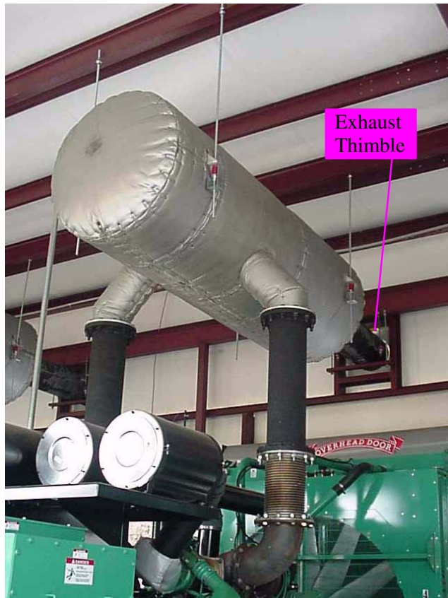
Figure 6-7: Generator Set Exhaust System Features. Dual Side Inlet Silencer, Flex Connectors, Exhaust Thimbles, and Mounting Hangers are Shown.
