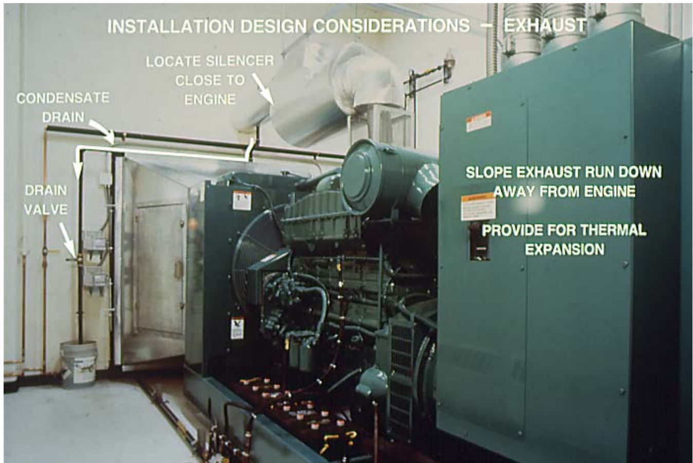
Figure 6-5: Typical Features of an Exhaust System for a Generator Installed Inside a Building.
