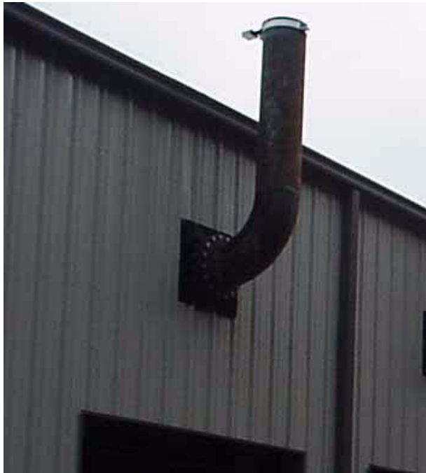
Figure 6–9. A Simple Exhaust System Fitted With a Rain Cap to Prevent Rain From Entering the Exhaust.
