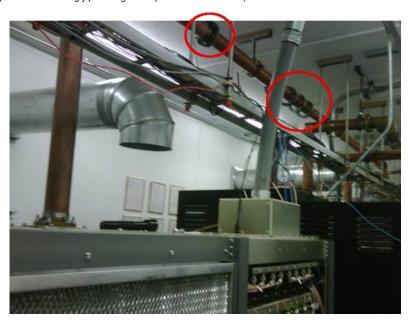
In the course of the installation, ferrites can and should be placed on pretty much every current carrying conductor – AC lines, remote control feeds, audio lines (don't forget the STL antenna cable). Nautel provides a handful with every transmitter that goes out the door, to ensure your installation isn't held up for want of some basic protection – talk to your sales rep if you think you need more.
