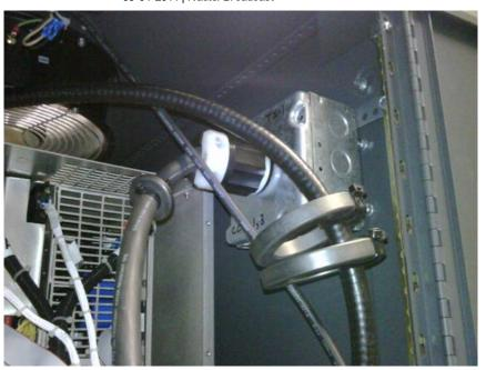
The above photo is a 1 kW AM transmitter installation – showing ferrite on both the AC and the coaxial cable... ultimately, for the purpose of common mode protection (trying to keep feed and return currents equal), size and permeability are somewhat less important than if we were making a choking by wrapping a single conductor around the toroid.
