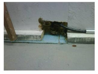
Further sleuthing showed a bit of a ground loop, in that the conduit carrying the electrical ground from the service panel to the transmitter ground strap was bolted to the transmitter chassis, creating a ground loop (the ground stud on the transmitter is insulated from chassis to provide a single point ground connection at the coaxial connector – the stud is connected to the coax connector via 2 AWG wires).
