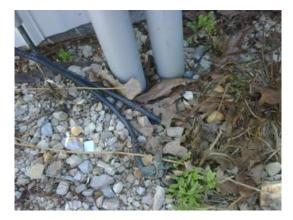
What you see in the above picture is indeed a ground rod. It was approximately two feet long and driven into the ground at about a 60 degree angle, so the far end was maybe a foot under ground – it could easily be wiggled loose by hand. In short, the best path to dissipate a lightning strike was through the transmitter power supplies to the AC lines.
