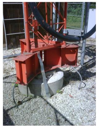
Unfortunately, the one thing we didn't see anywhere between the tower and the transmitter, after checking the strap, was a ground rod... effectively, the tower was connected directly to the transmitter. At that point, we decided to further investigate the AC entrance ground, which was the only path to ground for lighting, besides through the transmitter power supplies. We found this...
