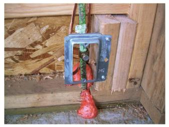
3. The foundation has been poured, the walls have been framed and the rebar electrode can be seen protruding through the mud sill. The electrician has sealed the hole around the electrode. The acorn clamp and the #4 AWG grounding wire coming from the panel have been connected to the rebar electrode.
