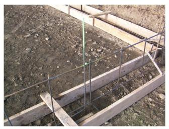
1.Installation of an approved electrode: The footing forms and the required rebar steel are set, and the top of the #4 rebar that will serve as the electrode has been painted bright green. This identifies the electrode location for the electrician and also allows the code inspector to inspect the electrode installation.
