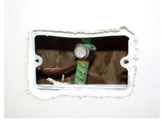
7. After the drywall is installed, the mud ring provides satisfactory access for visual inspection of the grounding assembly. A blank plate will cover the mud ring.
