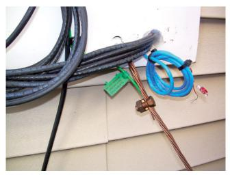
6. The other #4 AWG is used to ground the cable TV and phone service. The cable TV has been bonded, but the phone service box has not been installed yet.
