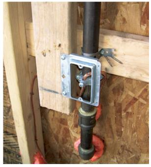
5. One of the #4 AWG wires is used to bond the gas line coming from the meter. Note the mud ring, which allows access for inspecting the bond.
