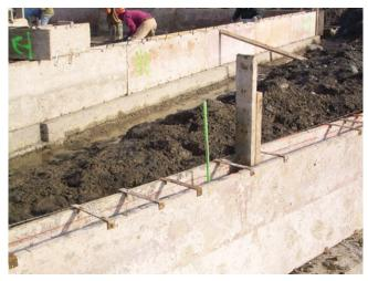
2.The formwork is complete and the spray-painted electrode can be seen protruding above the form panel. The location of the electrode is determined by the proposed location of the entrance conductors and the home's service panel.
