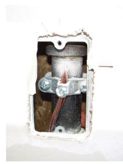
8. The bonded gas line from picture 5 is pictured with the finished drywall. A blank plate will cover the mud ring.
