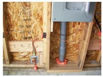
4. The panel has been installed. The #4 AWG wire is connected to the rebar electrode. Note the various runs of #4 AWG that will be used to bond the gas line, water lines, cable TV, phone service, etc.
